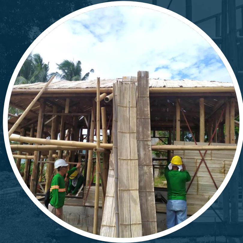
FLATTENED BAMBOO INSTALLATION
